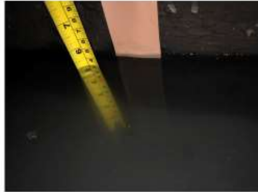
Water testing after application
